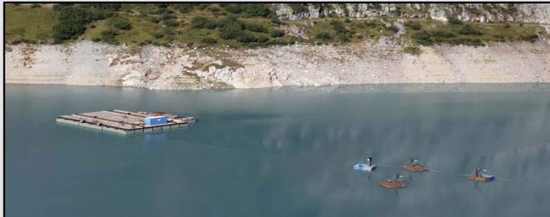
Lower intake floated into its final position
