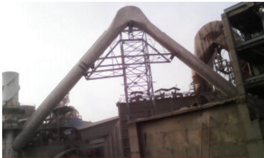
Figure 20: Hot air recirculation from stack to cooler
